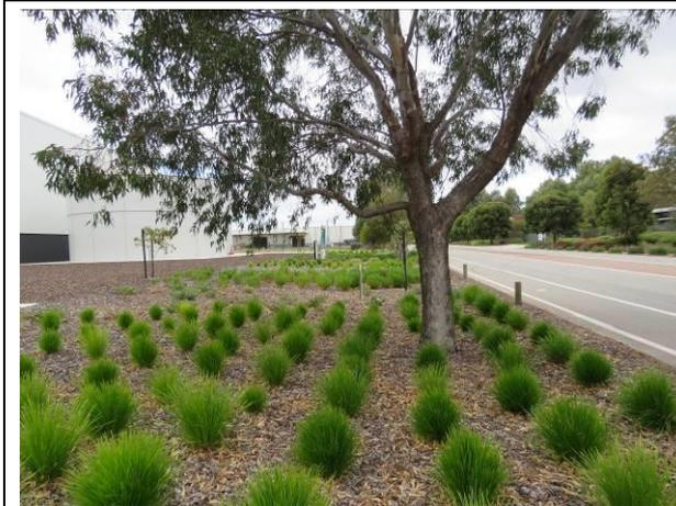
Note absence of roadside kerb/edging to allow for stormwater drainage from road, Marriott Road.
