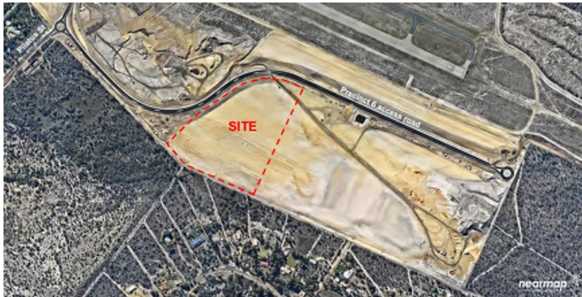
Figure 2 : Precinct 6 access road (June 2017)
