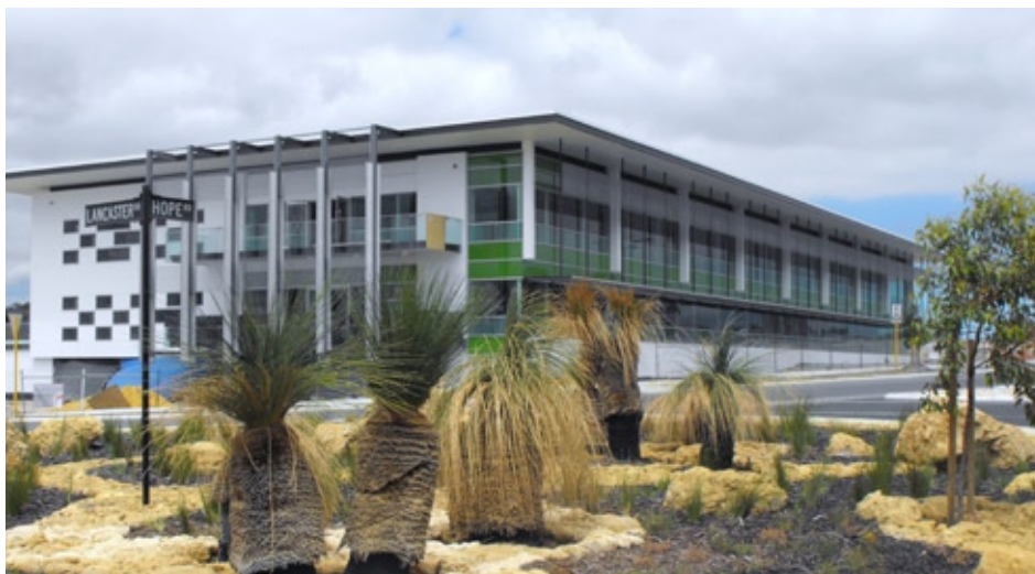
7 Hope Road, Jandakot City Office Park
